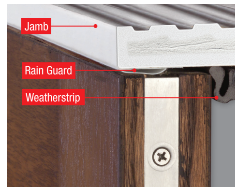
Top of door; exterior view.
